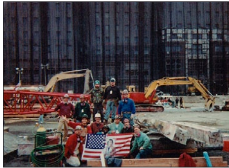
Ironworkers at Ground Zero
